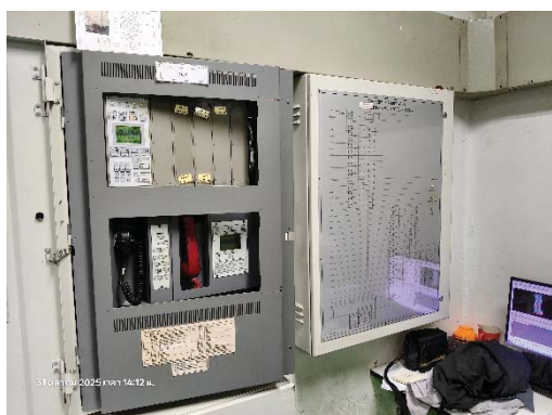
Fire Alarm Control Panel : FCP
